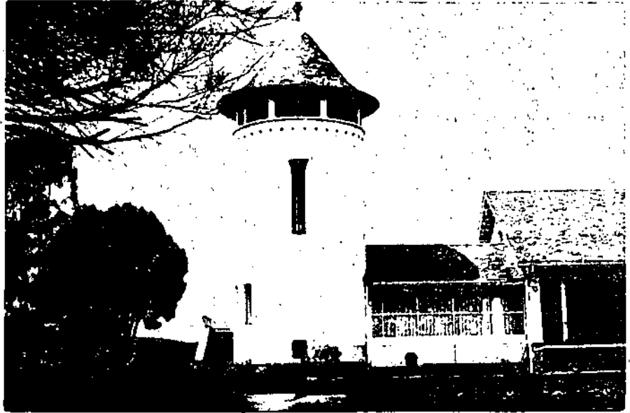
Observation Tower at La Rochelle
